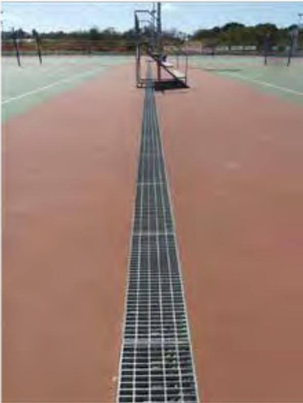
The large dish drain between the courts is located outside of the runoff area and does not present a trip hazard to either players or spectators. The distances between the court sidelines at this facility are either 6.10 or 9.00m. At 9.00m the wider separations provide plenty of space for seating, shelters, and future-proof the courts for the addition of covered roof structures at a later date.
